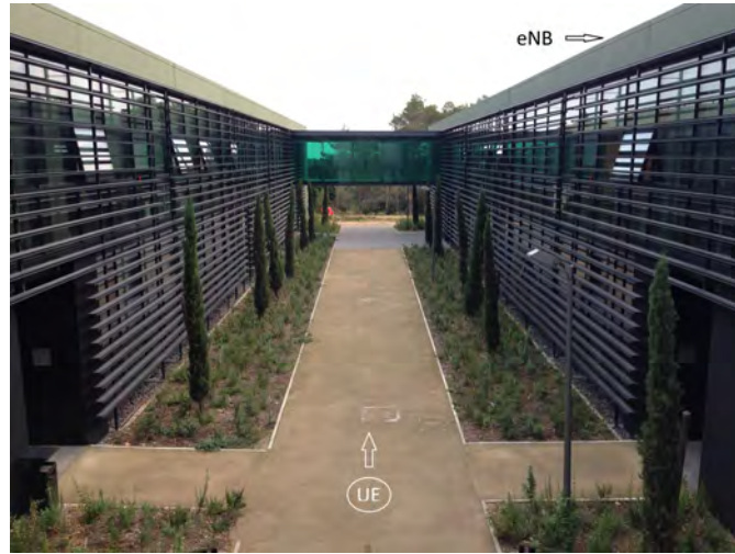
Figure 5.11: NLOS environment with eNB on the roof of left building
