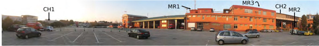
Figure 2.15: Five node mesh network trial in Bellaterra, Spain. MR1 is located at the roof of the red fire brigade building. CH1 and MR2 are located on opposite sides of the parking lot in front of the building. CH2 and MR3 are on the other side of the building.
